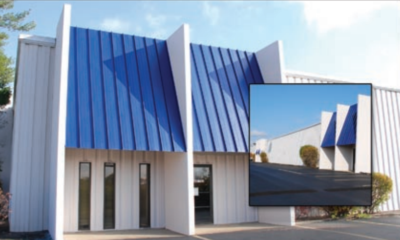
...Puritas Business Centre I 4455-4505 & 4517-4521 West Parkway, Cleveland, Ohio
