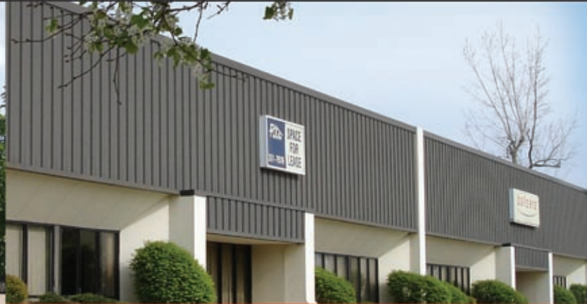
...Brunswick Business Centre III & IV 1126 & 1130 Industrial Parkway
