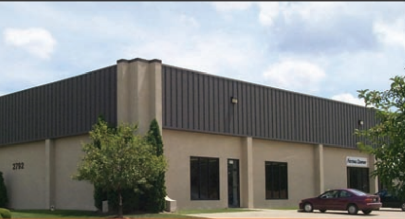
...Brunswick Business Centre I & II 2774 & 2792 Nationwide Parkway
